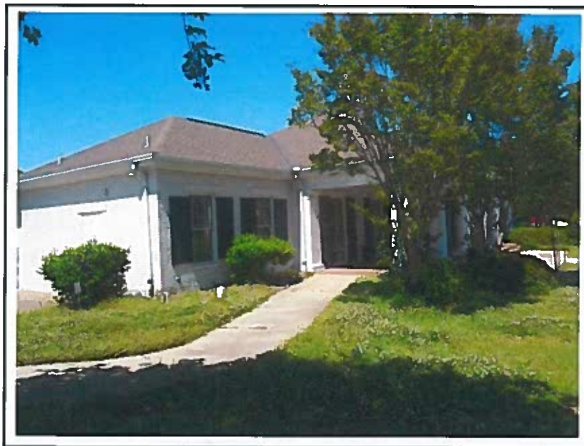
2. VIEW OF THE SOUTHWEST AND SOUTHEAST ELEVATIONS OF THE BUILDING. DATE TAKEN: April 15, 2018
