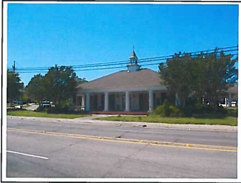
1. VIEW OF THE SOUTHEAST ELEVATION OF THE BUILDING. DATE TAKEN: April 15, 2018
