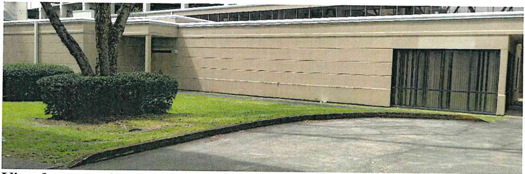
View from east facing west.
