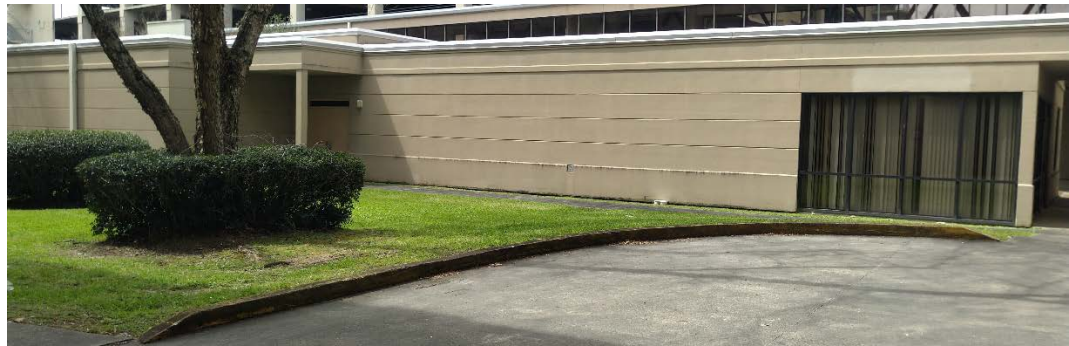
View from east facing west.
