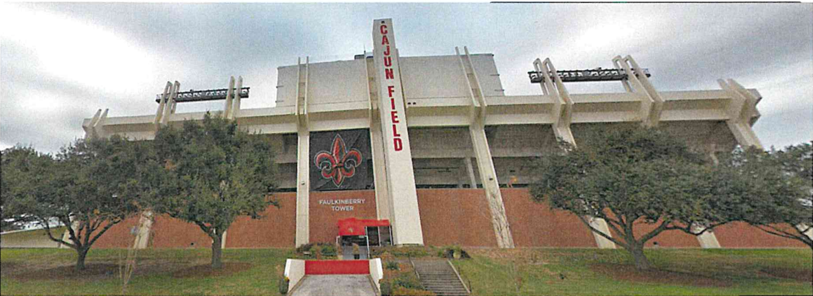
View from west facing east.
